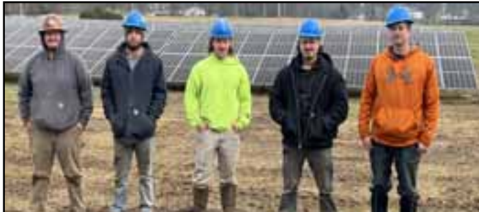
Thoroughbred Construction at Moraine State Park Solar Project L to R: Brad Nelson, David Mospan, Ian McElroy, Matt Brestensky & Zak Bykowski
