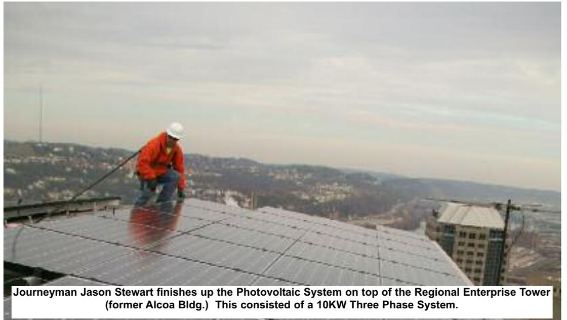
Journeyman Jason Stewart finishes up the Photovoltaic System on top of the Regional Enterprise Tower (former Alcoa Bldg.) This consisted of a 10KW Three Phase System.
